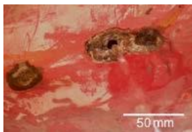
Figure 4. Fault example from a segment of a pipeline induced by punctured hole [2].
