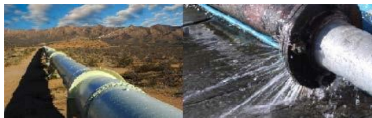
Figure 1. Picture of a pipeline crude oil transportation system with failure example [1]
